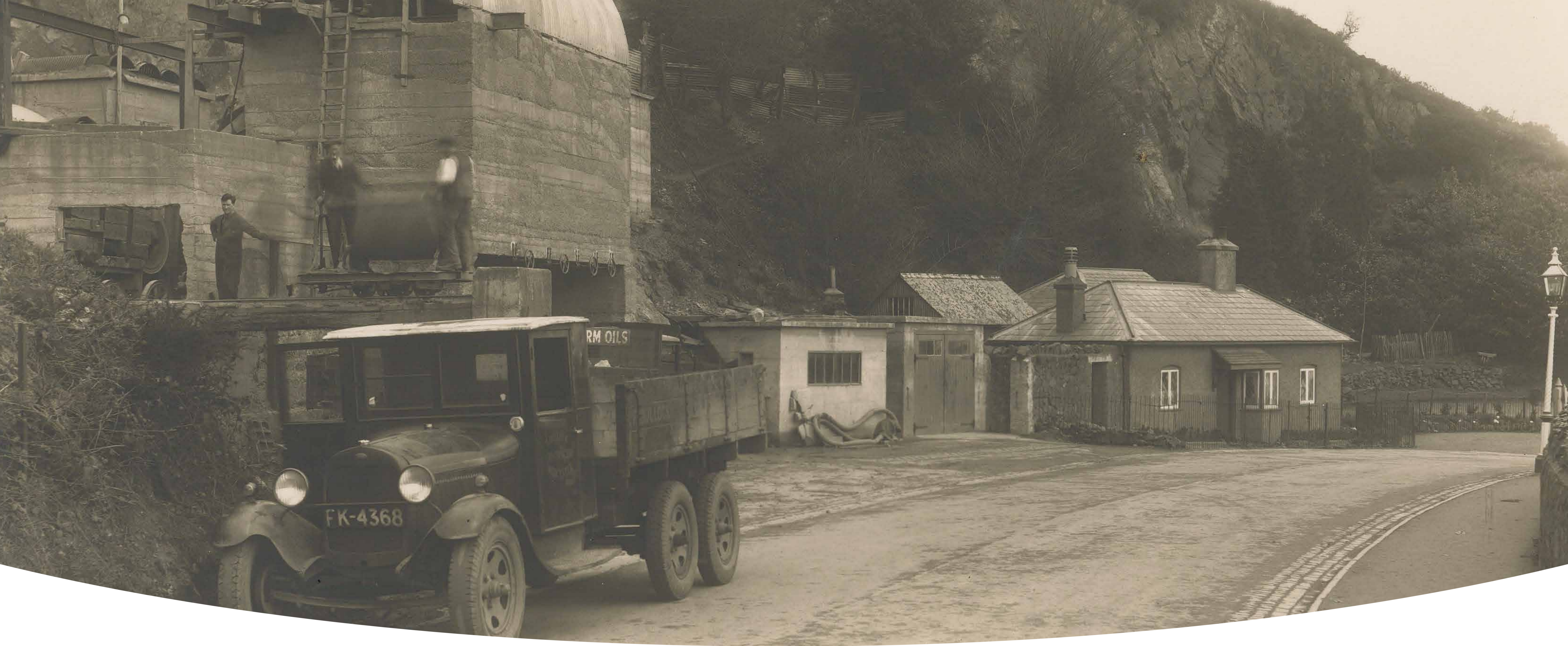
Quarry buildings and equipment at Earnslaw Quarry (c1930)
