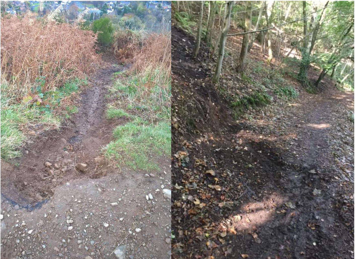
Path damage caused by wild trails to legitimate paths. Left – path cut away at the entrance to a trail. Right – fanned material at trail exit. Malvern Hills.
