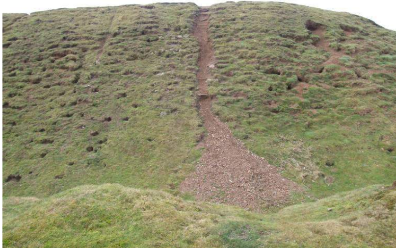
Figure 18: Gullying and outwash on the ring-work caused by water erosion.
