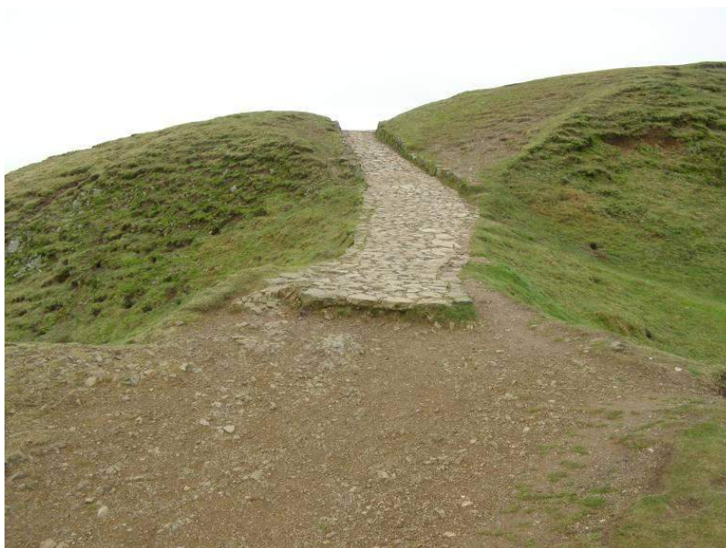
Figure 19: Path erosion where the paved path meets an un-surfaced area.
